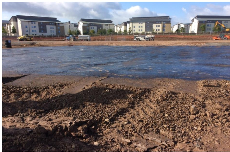
Soil Stabilisation - Bitumen
