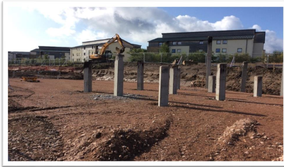
Energy Centre - Piles
