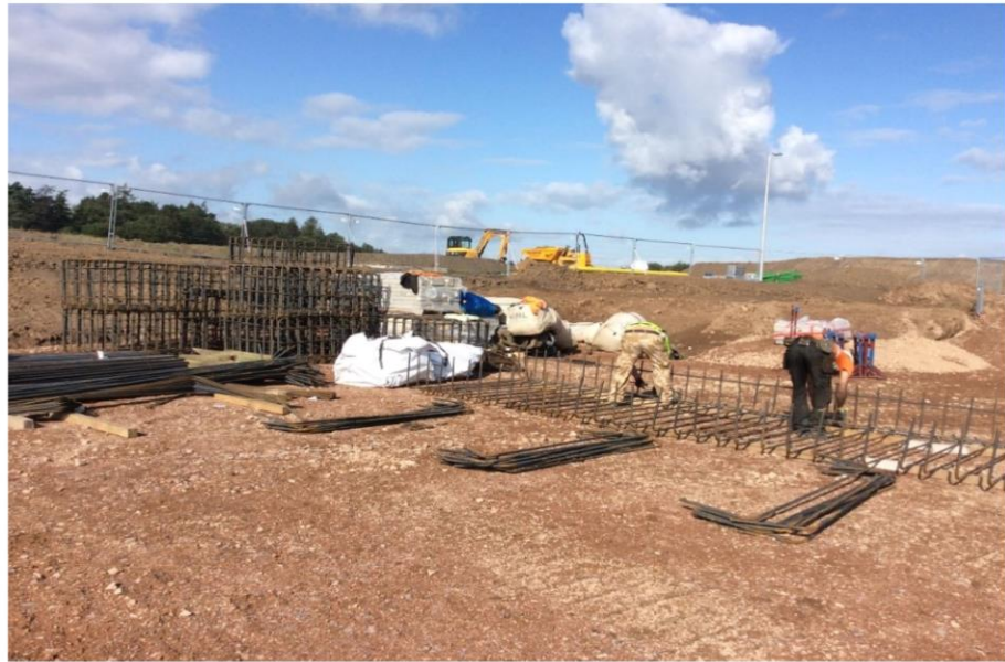
Energy Centre – Steel Reinforcement
