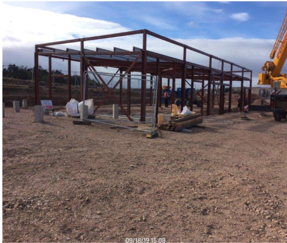
Energy Centre - Steelwork
